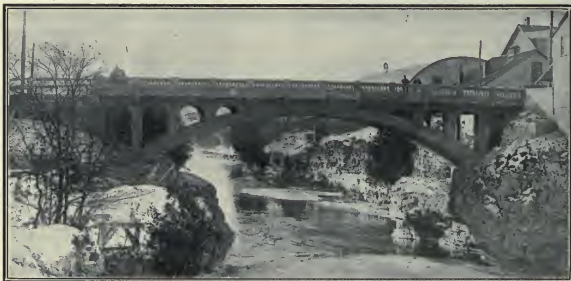
Tower Street Bridge, Fergus, Ont.
